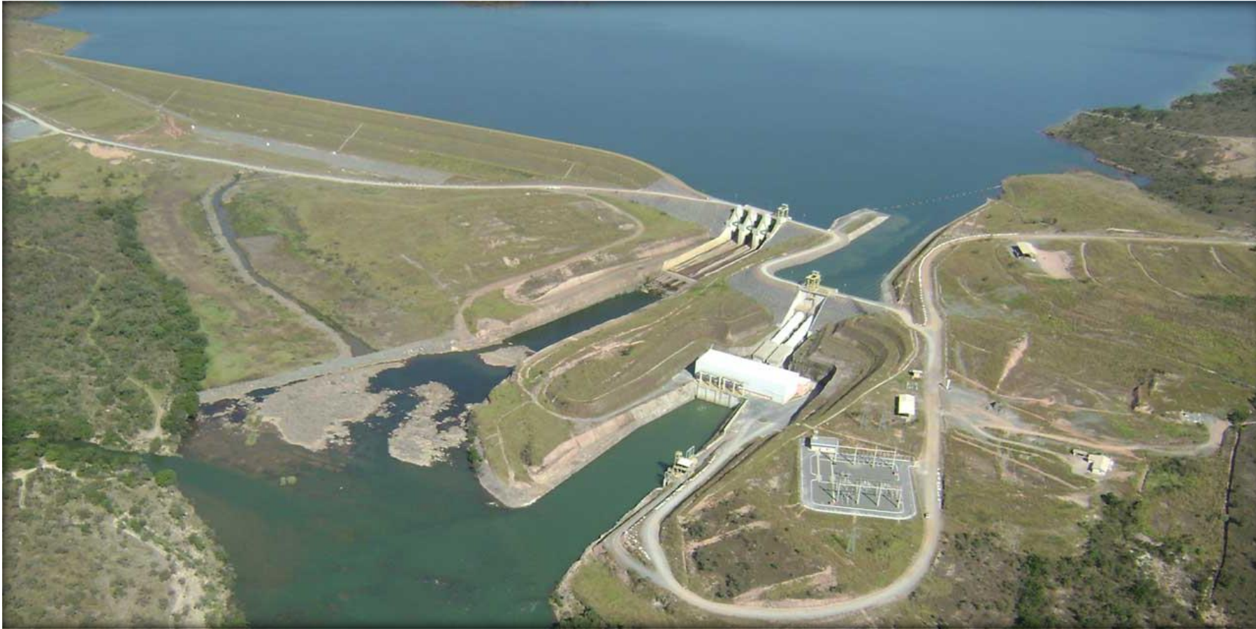
Hydro Power Plant
